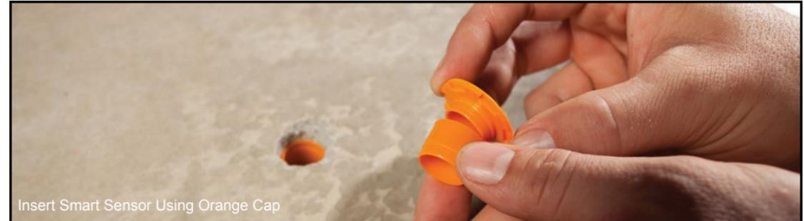
Insert Smart Sensor Using Orange Cap
